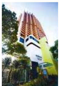
Somerset Liang Court Property
