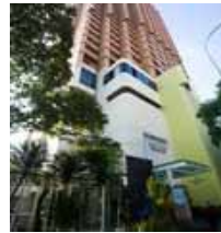
Somerset Liang Court Property
