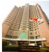
Somerset Olympic Tower Property Tianjin
